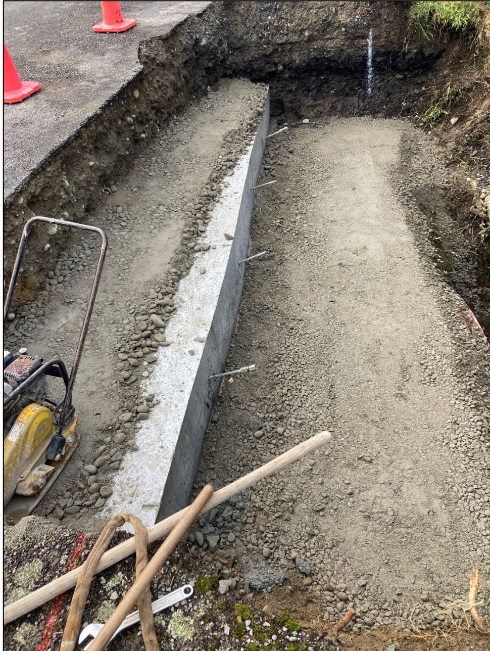
Figure 4: Herd Street culvert head wall works underway
