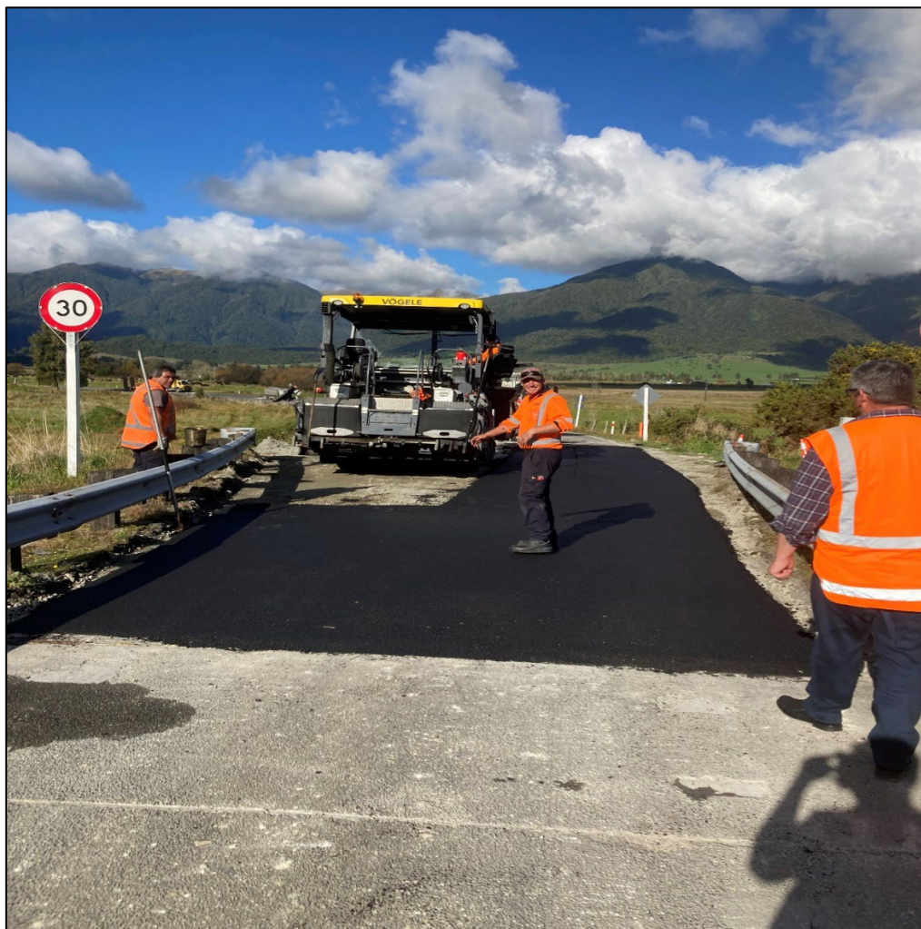
Figure 5: Sealing works for Crooked River No.2 bridge approaches
