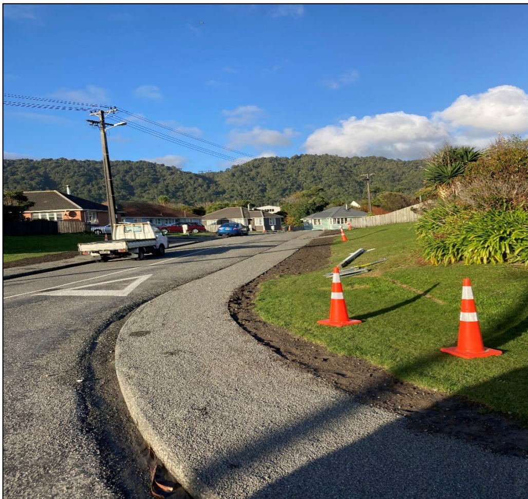
Figure 2: McKane Place footpath works completed.
