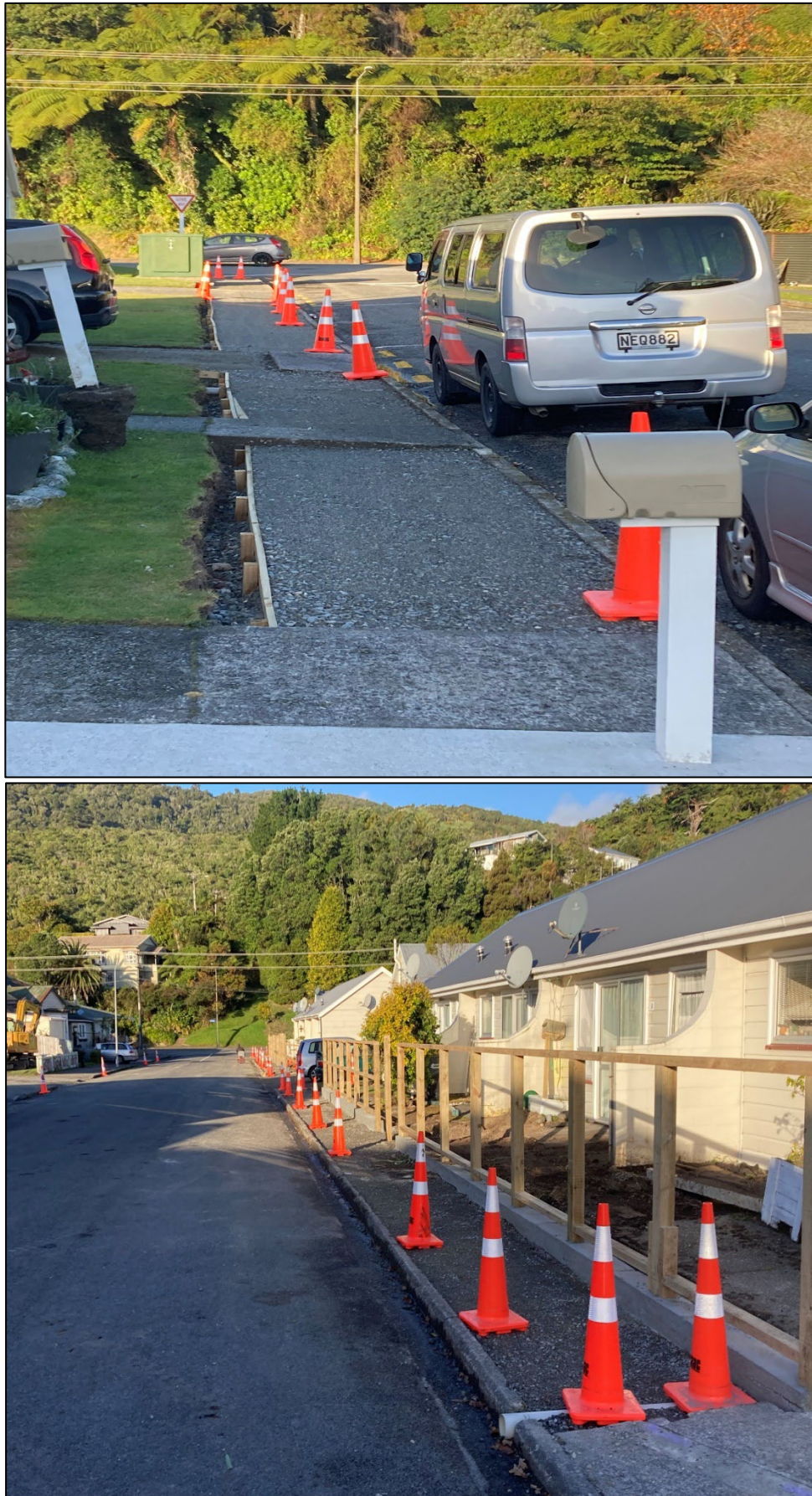
Figure 1: Ngarimu St and Fricleton St renewals underway
