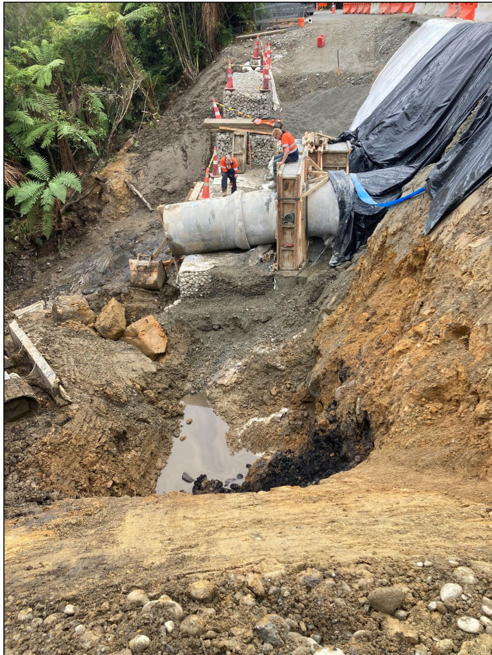
Figure 3: New culvert pipe installed and gabions in place
