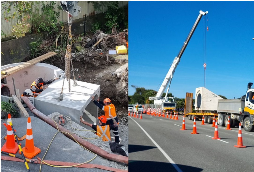
Figure 9 - Tasman Street Stormwater Upgrade
