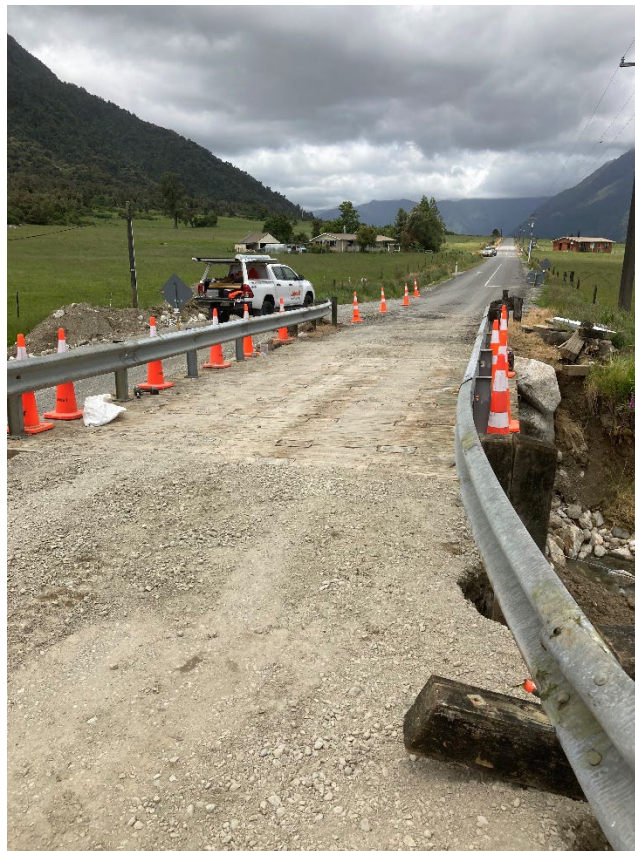
Figure 3: Clear Creek Bridge Replacement on Site Work before Christmas 2023
