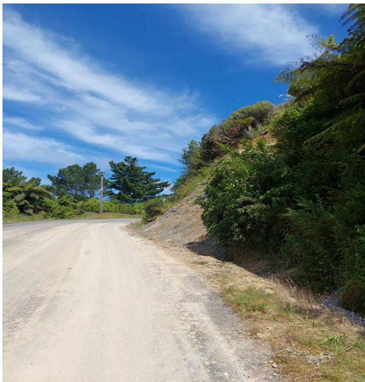
Figure 7- Tasman View Slip Remedial Work
