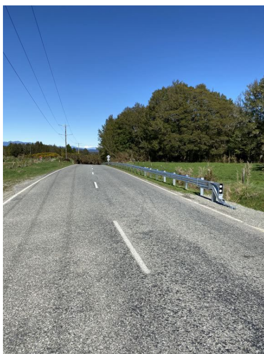
Figure 4: Guardrail Barrier installed at Atarau Road
