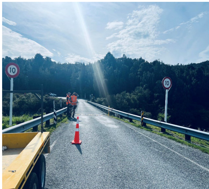
Figure 6: Temporary Installation of The Speed Humps at Crooked River Nos 2 Bridge
