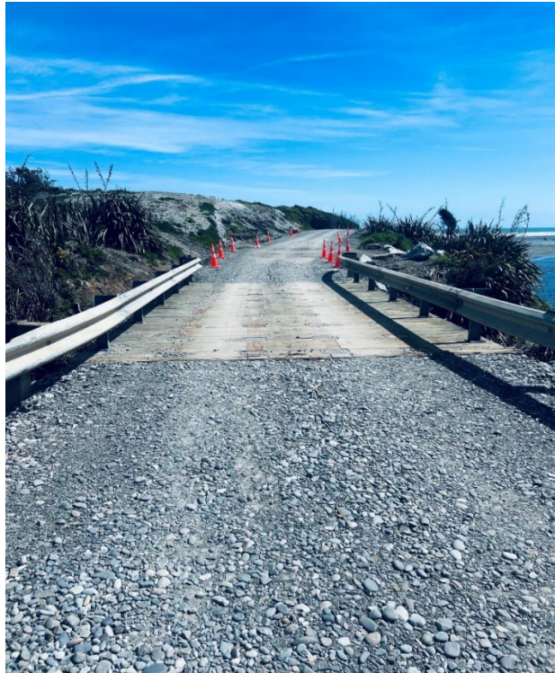
Figure 2: Seven Mile Bridge
