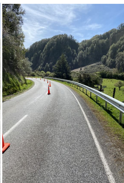
Figure 5: Guardrail Barrier installed at Nelson Creek Road
