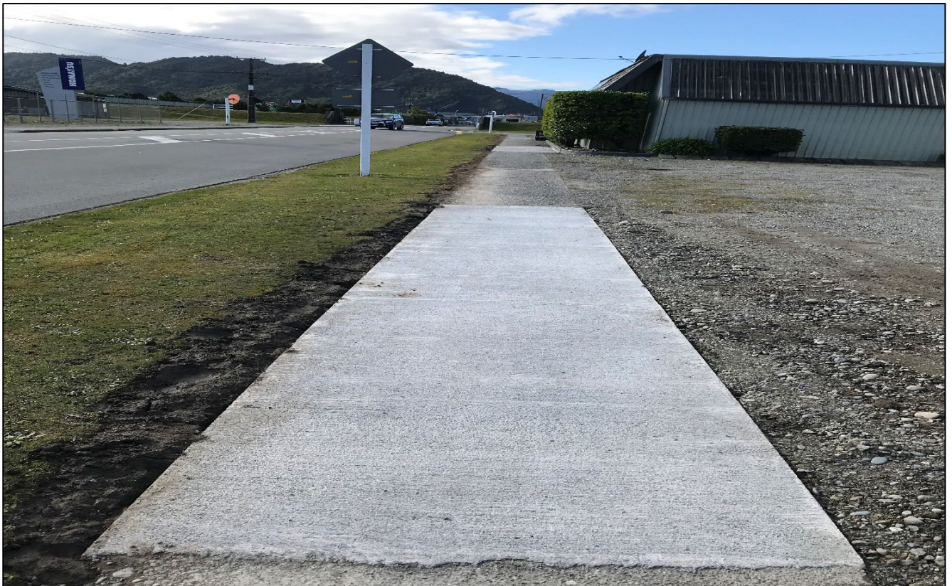
Figure 5: Footpath remedial works on Preston Road
