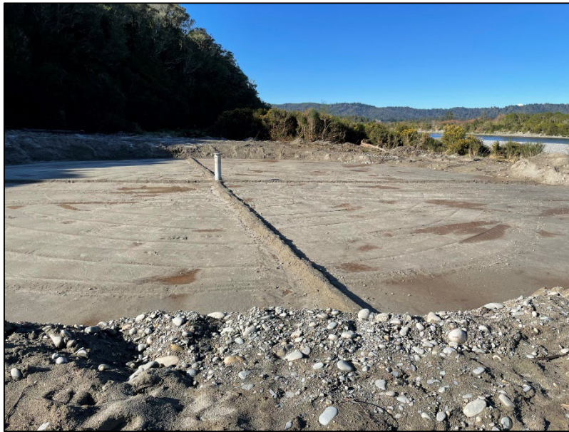
Figure 9: Bore # 4 Installation – Pre-liner Install.
