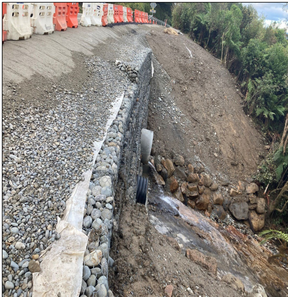
Figure 7: Taylorville Road – Retaining Wall
