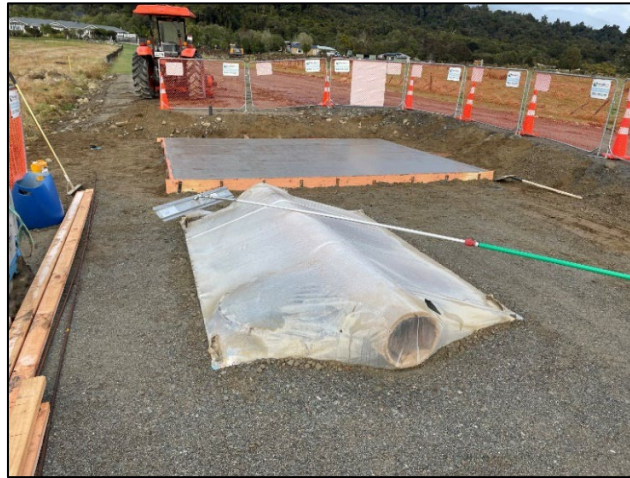
Figure 13: Dry Vault and Toilet Pad
