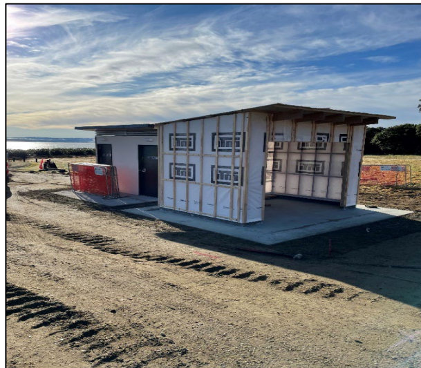
Figure 14: Completed Toilet and Shelter awaiting Cladding
