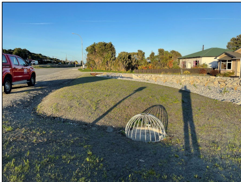
Figure 11: Tasman Street - Completed Landscaping Looking South.
