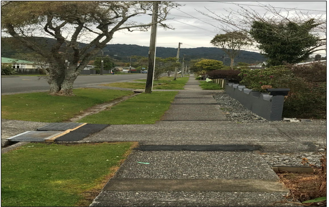
Figure 4: Footpath maintenance works on Marlborough Street
