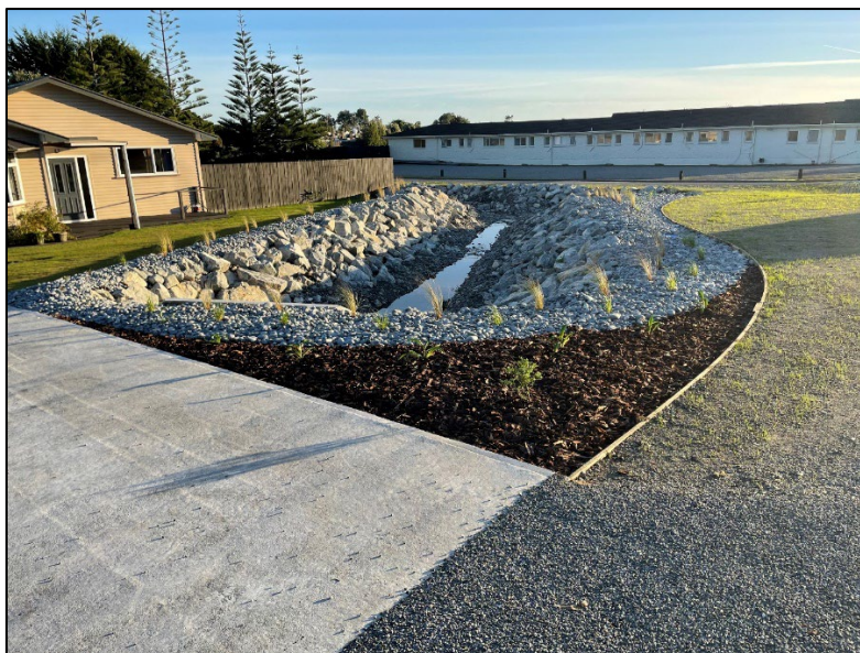
Figure 12: Tasman Street - Completed Landscaping Looking Northwest.
