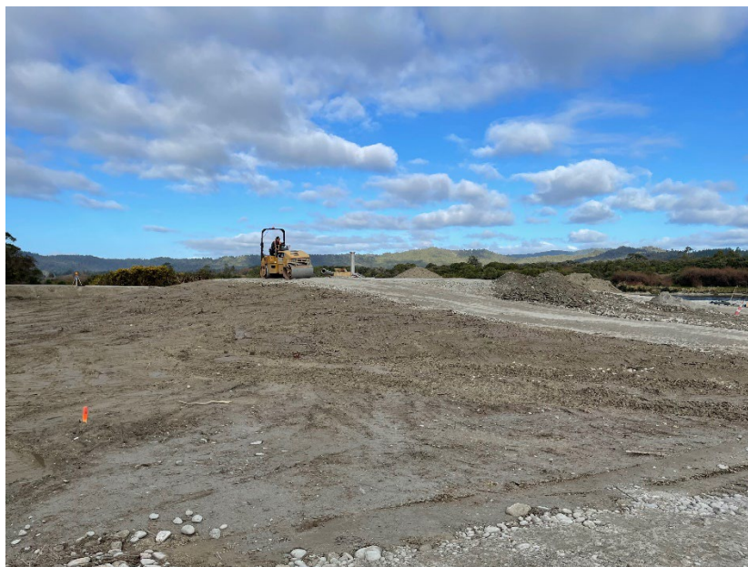
Figure 10: Bore # 4 Installation – Post Liner Install.
