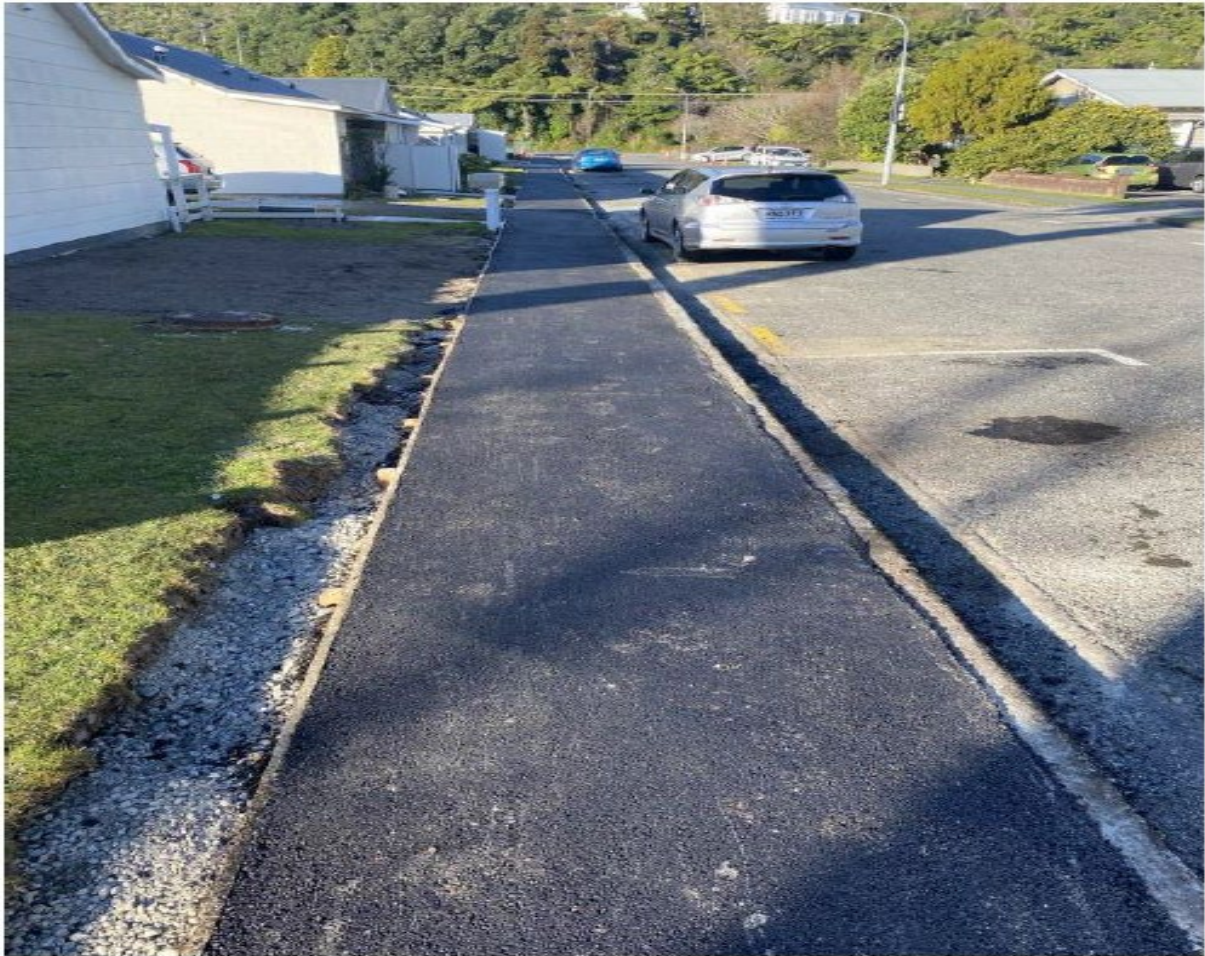
Figure 6: Footpath renewal works near retirement flats on Ngarimu Street
