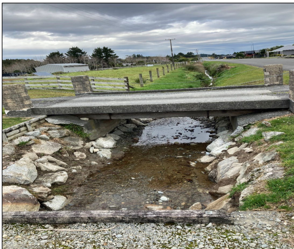
Figure 1: Drainage works on Coulson Road
