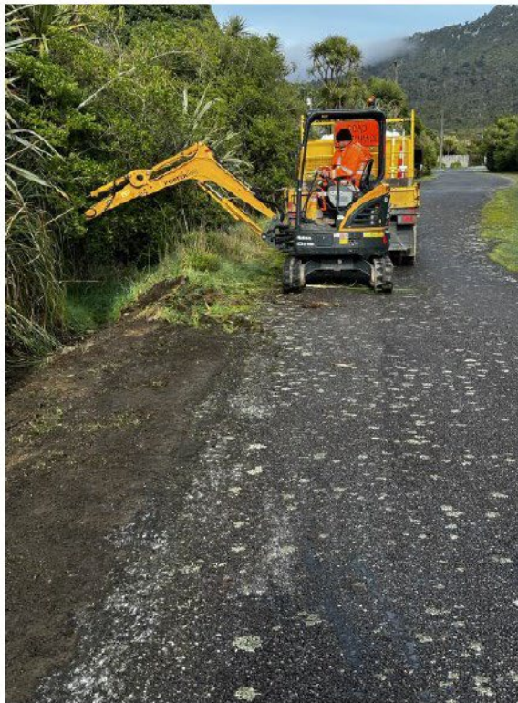
Fig 3 : Holland, Hawkin and Morpeth Street drain cleaning and shoulder flanking
