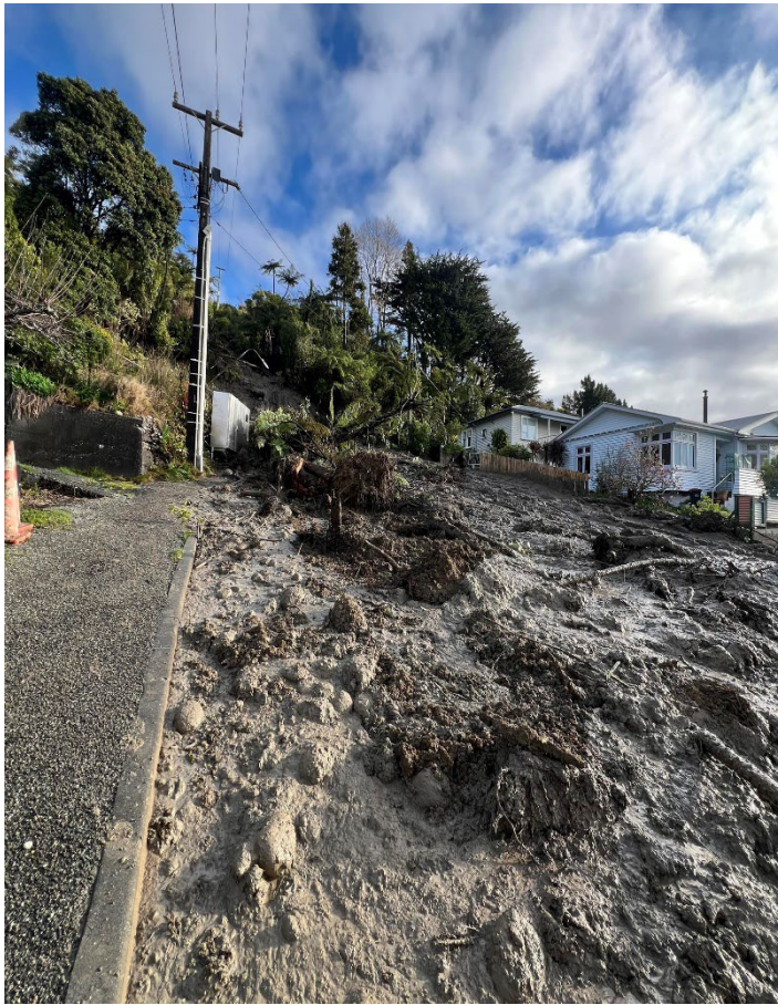
Fig 8: A second slip occurred at mid-day Monday 26 August
