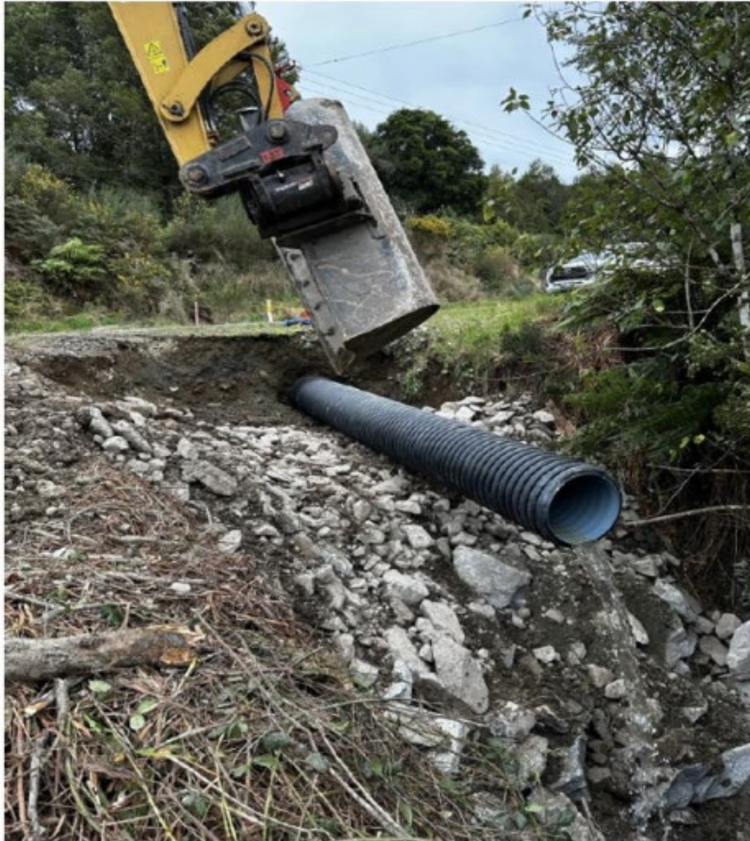
Fig 2 : Arnold Valley Road culvert reconstruction
