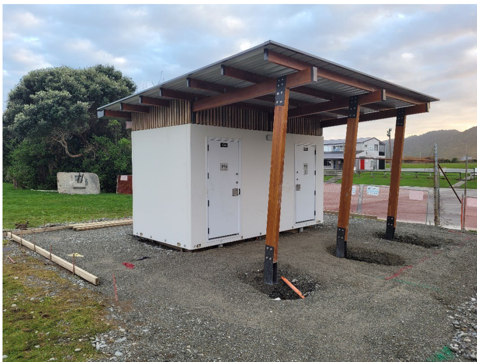
Fig 13: New Anzac Park Toilet Facility – under construction.
