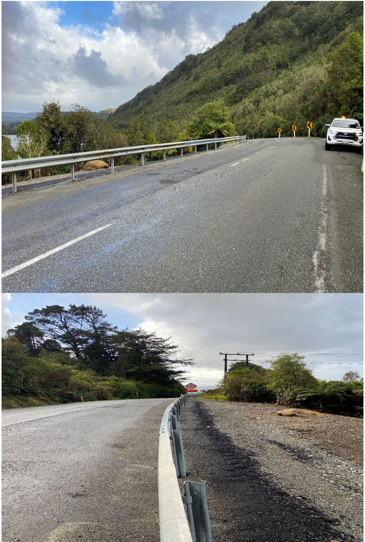
Fig 6: Taylorville road barrier works completed
