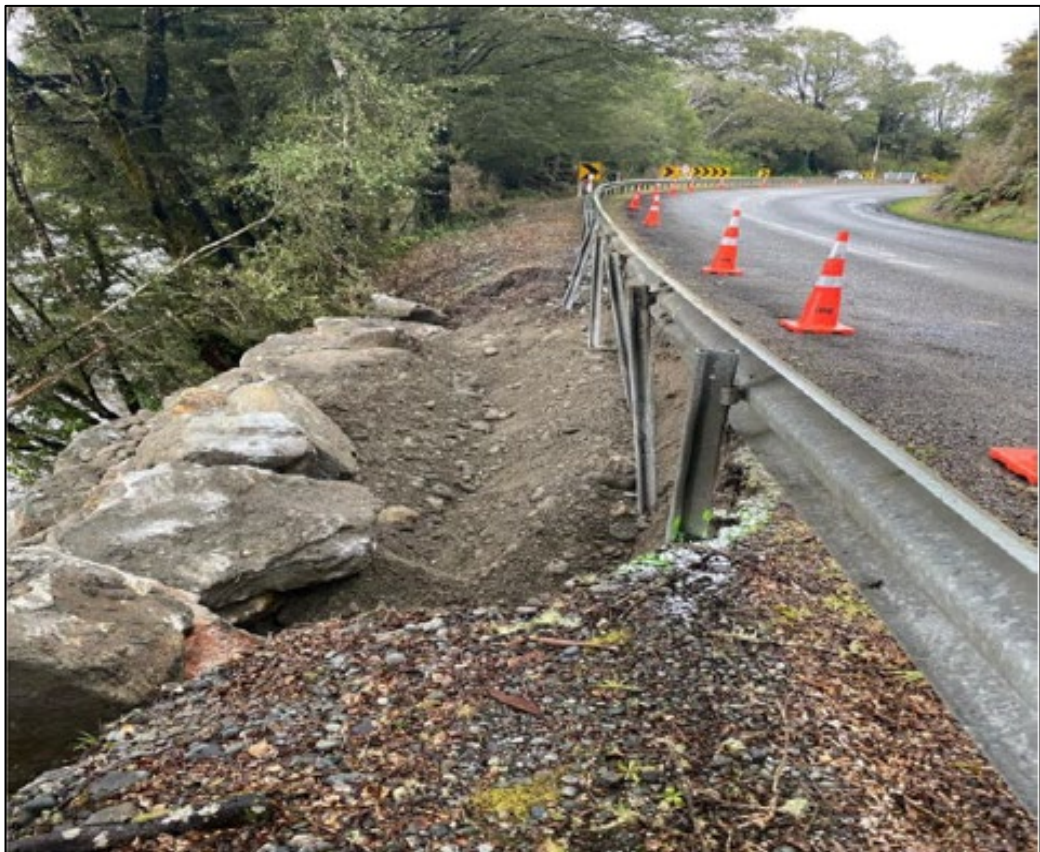
Fig 2: Slip on Taylorville- Blackball Road after remedial works
