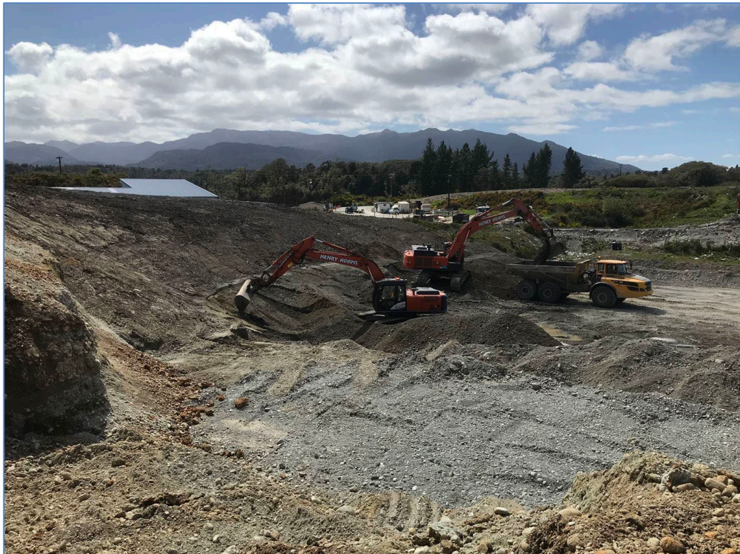
Figure 8: McLeans Pit Landfill Cell 3B Construction – Cell excavation looking north
