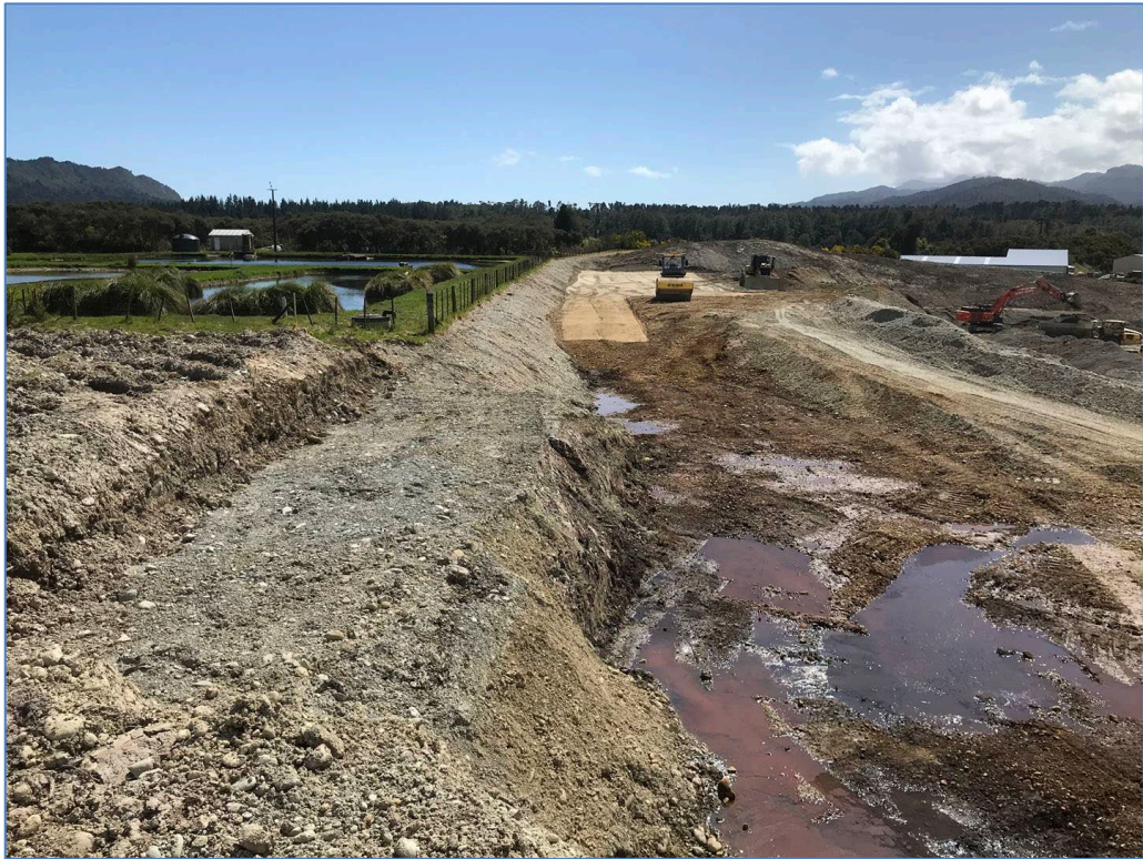
Figure 7: McLeans Pit Landfill Cell 3B – Western wall looking north
