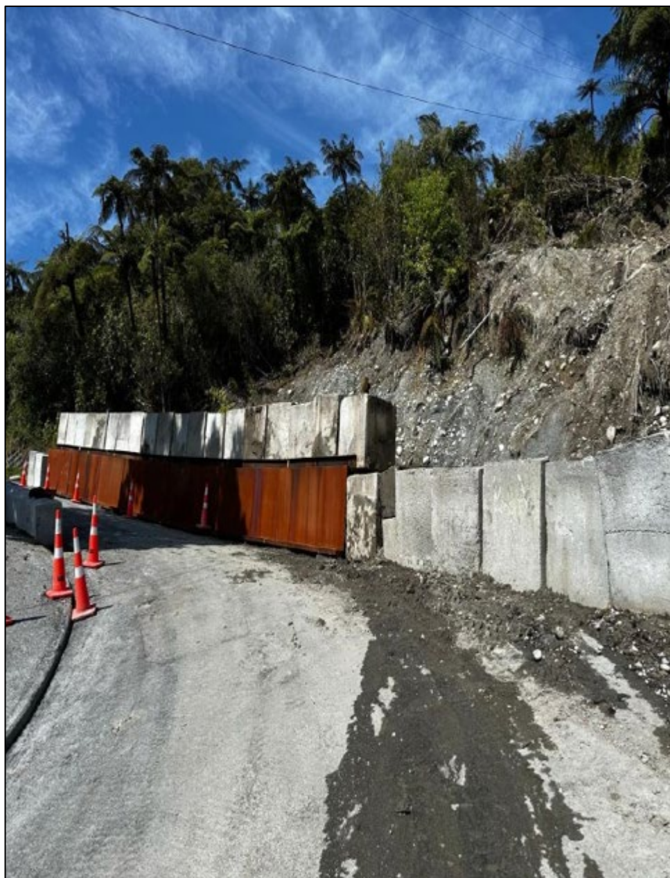
Fig 5: Milton Road temporary retaining wall strengthening works
