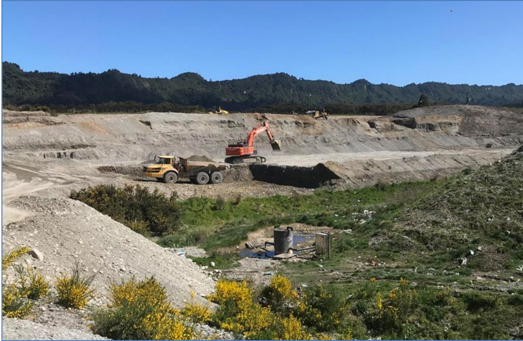
Figure 9: McLeans Pit Landfill Cell 3B Construction – Cell excavation looking west
