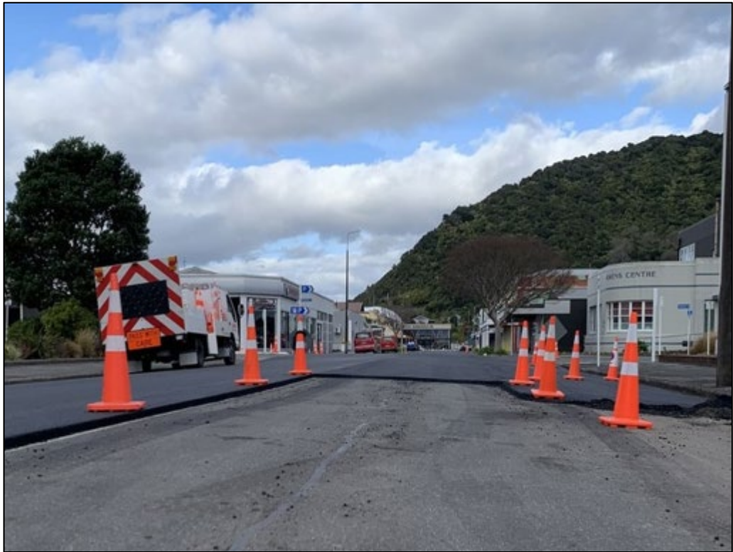
Fig 6: Re sealing works on Guinness Street
