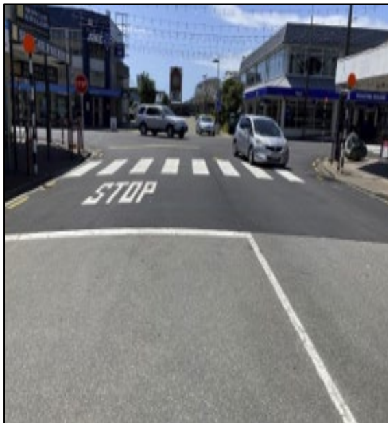
Fig 8: CBD Re-sealing and line marking works completed.
