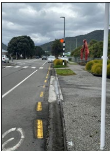
Fig 1: Kerb and channel cleanup work opposite Z pump Grey Highschool
