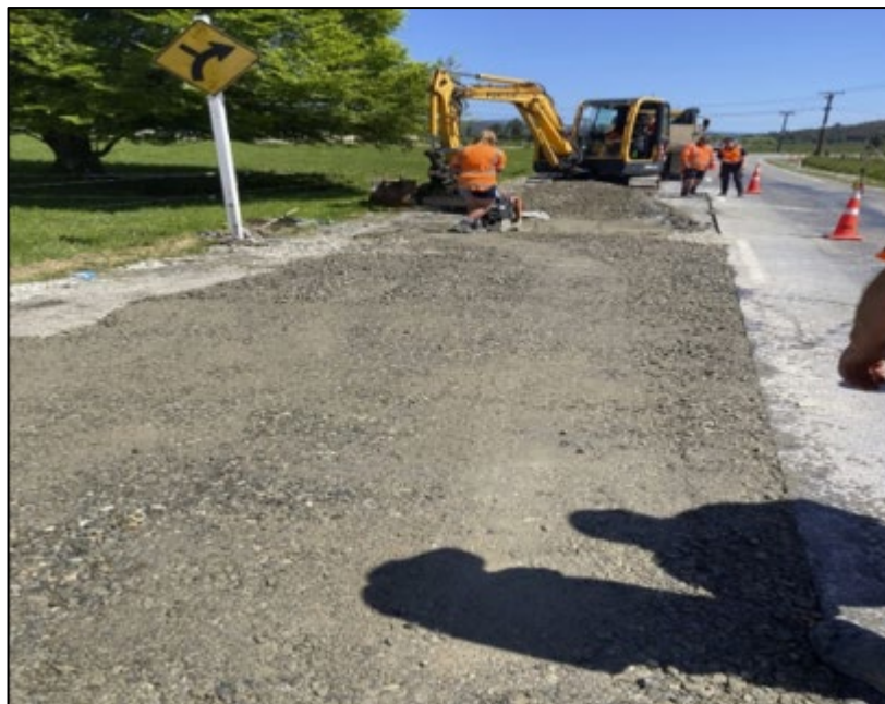
Fig 5: Dig out and reseal works at various locations of the district
