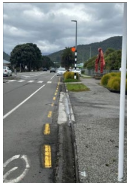
Fig 2: Kerb and channel cleanup works near
