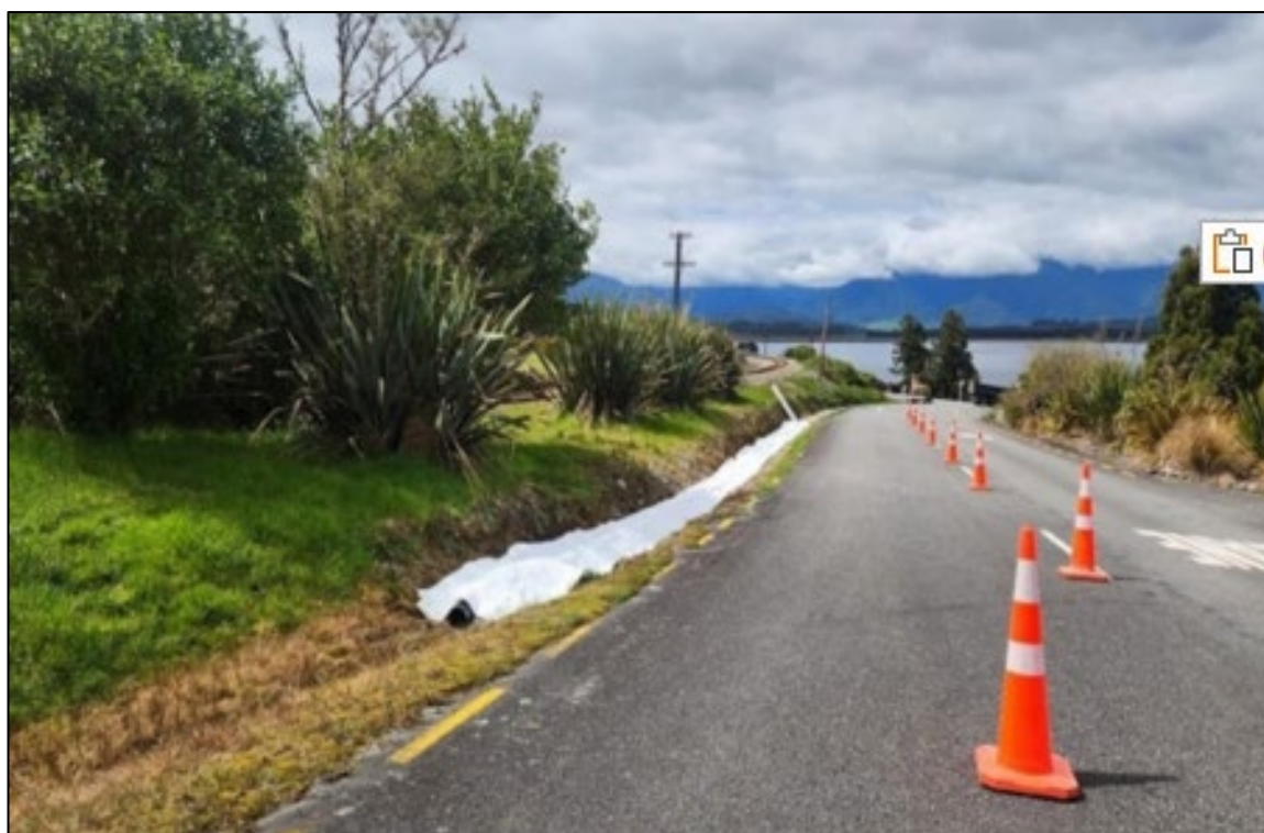
Fig 6: Existing open drain has been removed and a closed drain created.
