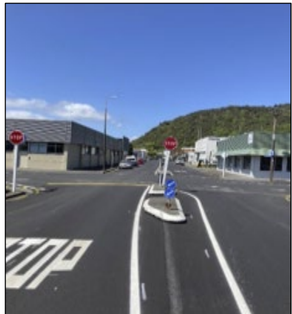
Fig 9: Final line marking works also completed.
