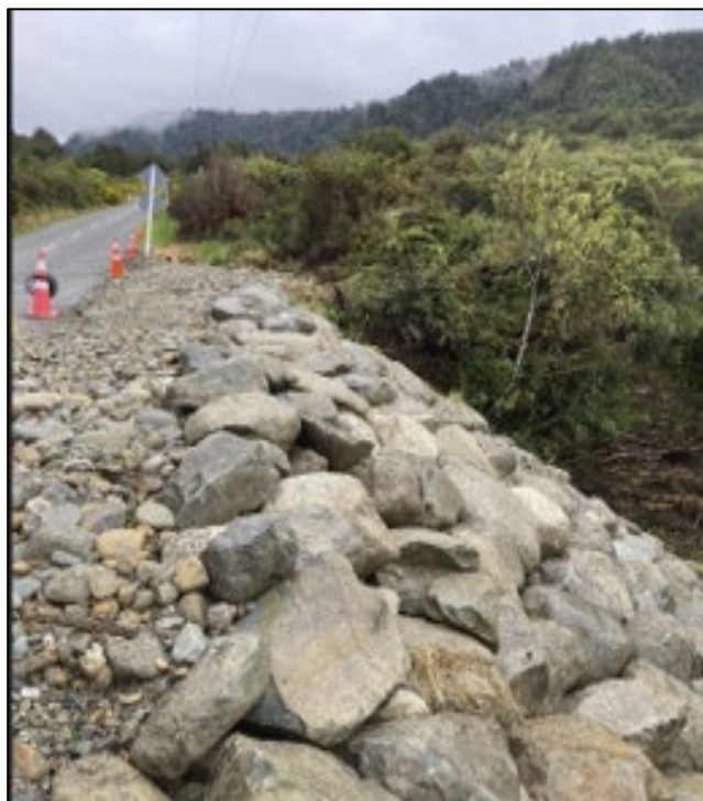
Fig 4: Slip rock protection works at Kumara-Inchbonnie Road
