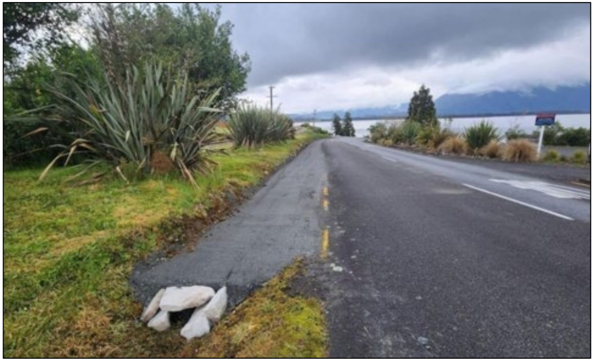
Fig 7: Drainage works completed and more parking spaces added
