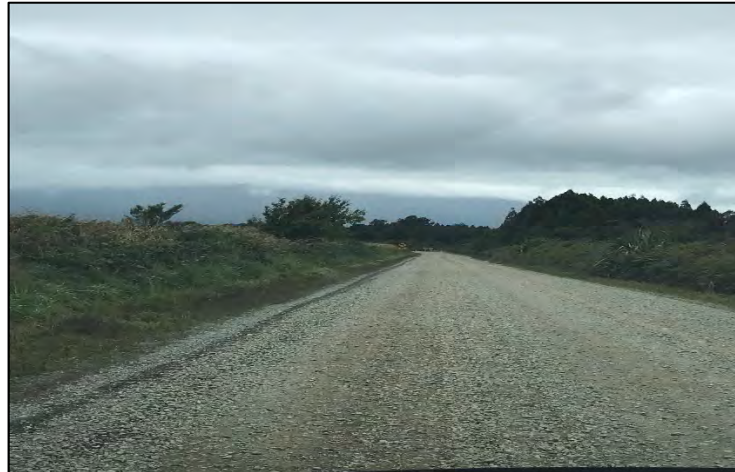
Fig 2: New gravel overlaid on Blairs Road, Grey District
