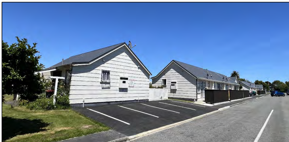
Fig 5: Ngarimu Street Roof Renewal work
