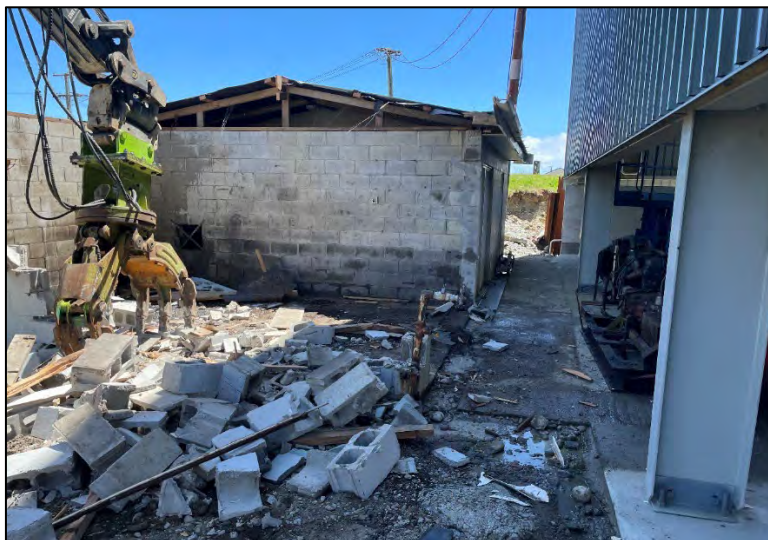
Fig 4: Demolition of Winch Shed
