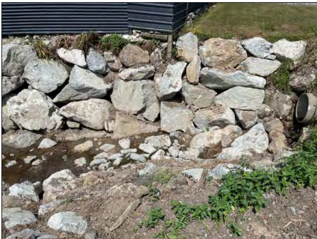
Fig 9: Oxford Street – rock protection work
