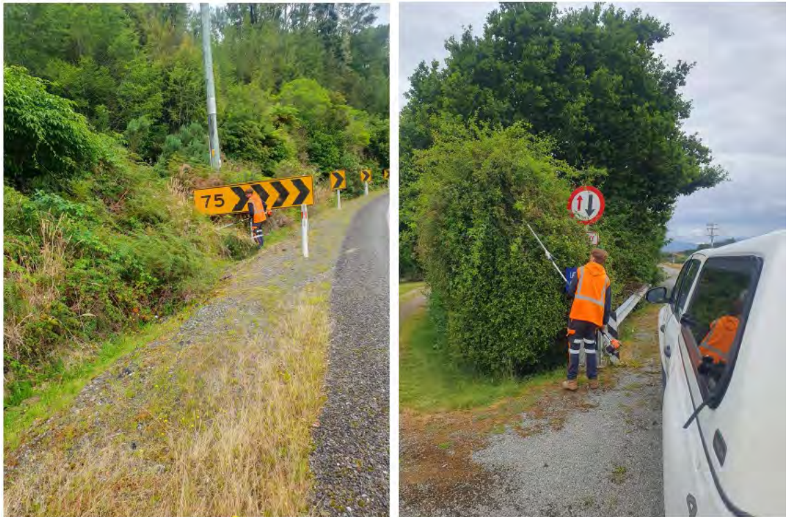
Fig 2: Vegetation Clearing works
