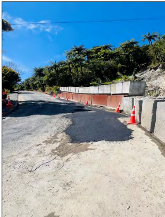
Fig 5: Temporary reinstatement works completed for the seal
