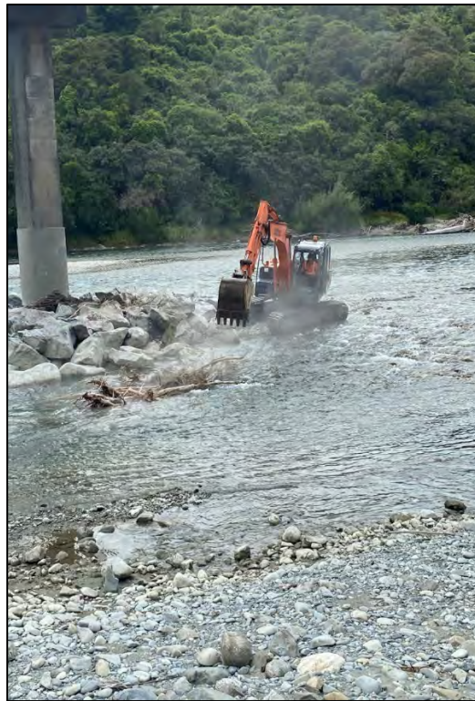
Fig 4: William Stewart bridge log removal works
