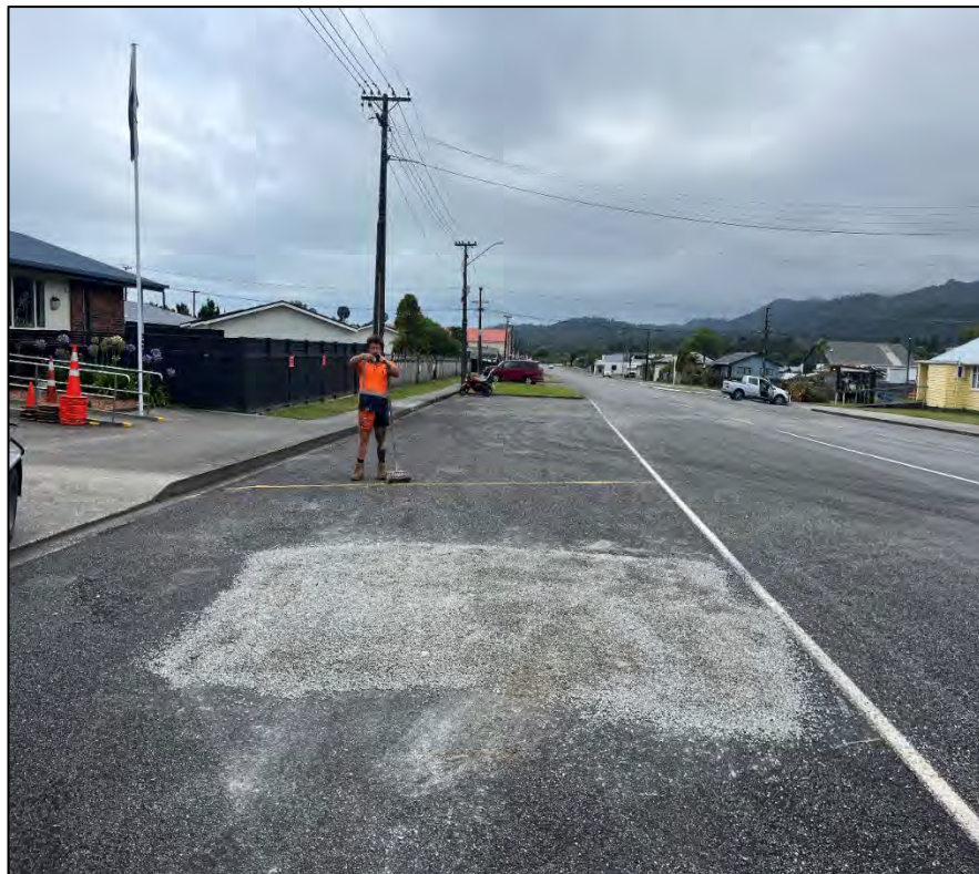
Fig 3: Seal Repairs in front of Runanga Fire Station
