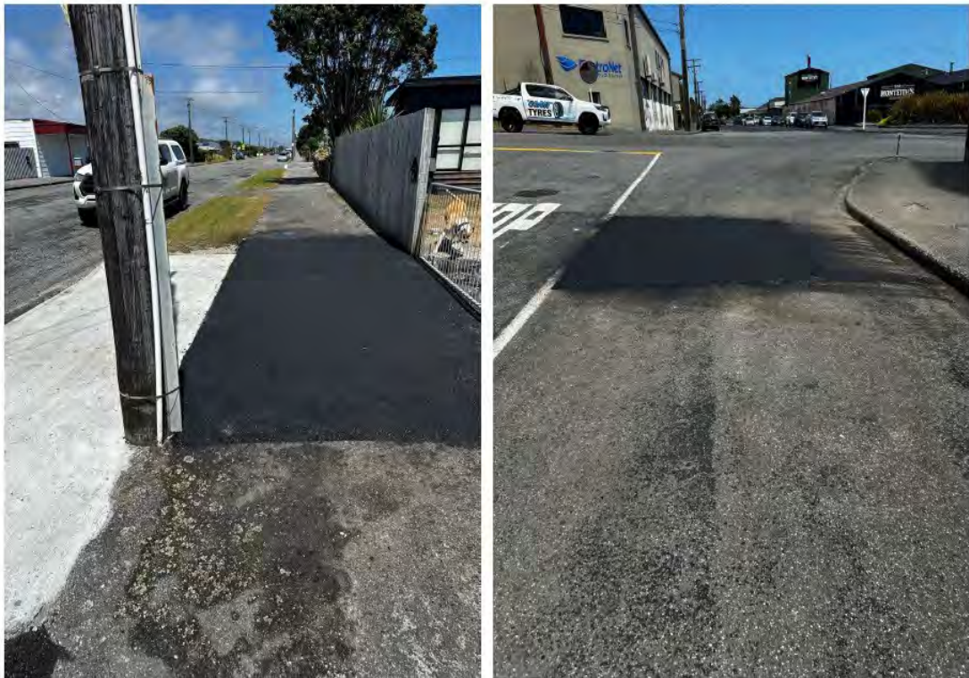
Fig 1: Asphalt repair works in Blaketown and Turumaha Street
