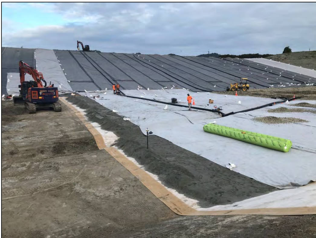
Fig 13: Photo showing the progression of liner layers being installed – looking northwest.
