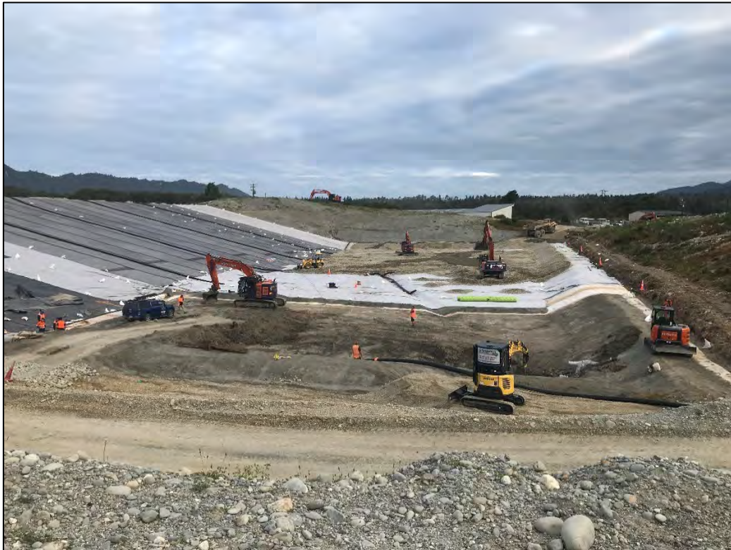
Fig 12: Photo showing the progression of liner layers being installed – looking north.
