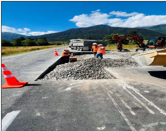
Fig 10: Lake Brunner Road pre-seal repair works
