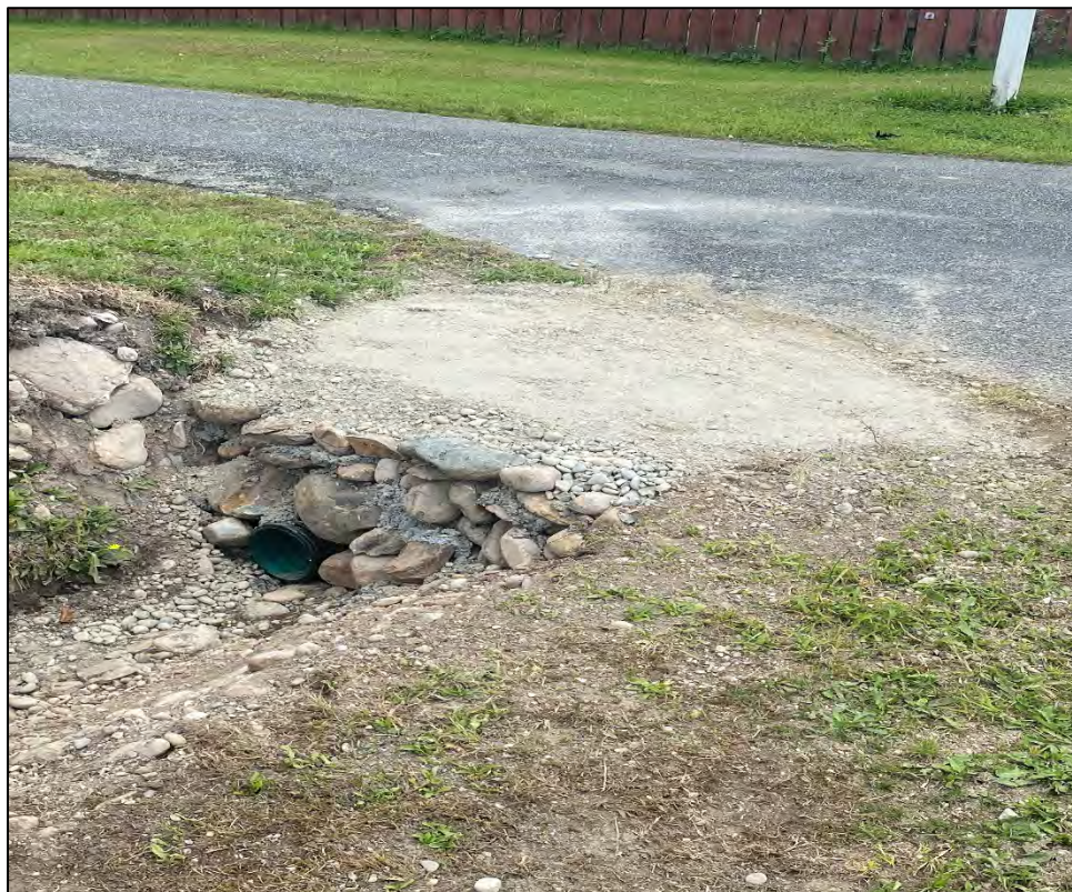
Figure 1: Culvert Extension on corner of Brodie and Deniston Street
