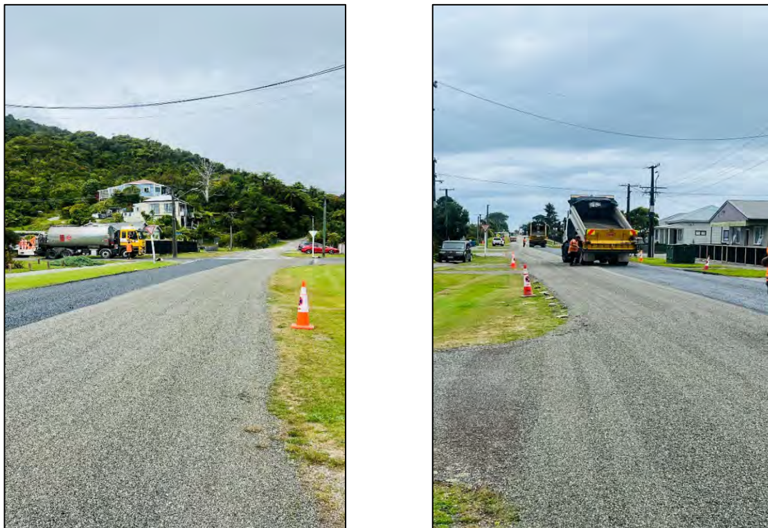
Figure 7 & 8: Resealing works in fox street Cobden
