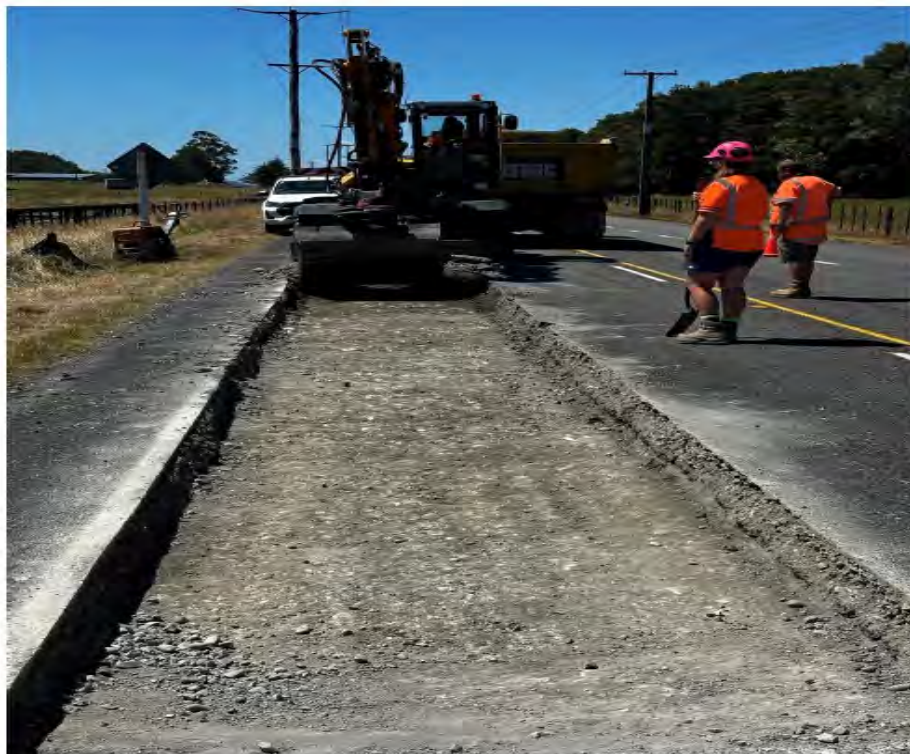
Figure 5: Pre-seal works on Lake Brunner Road
