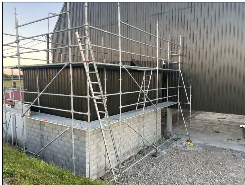
Figure 10: External View of New Winch Building
