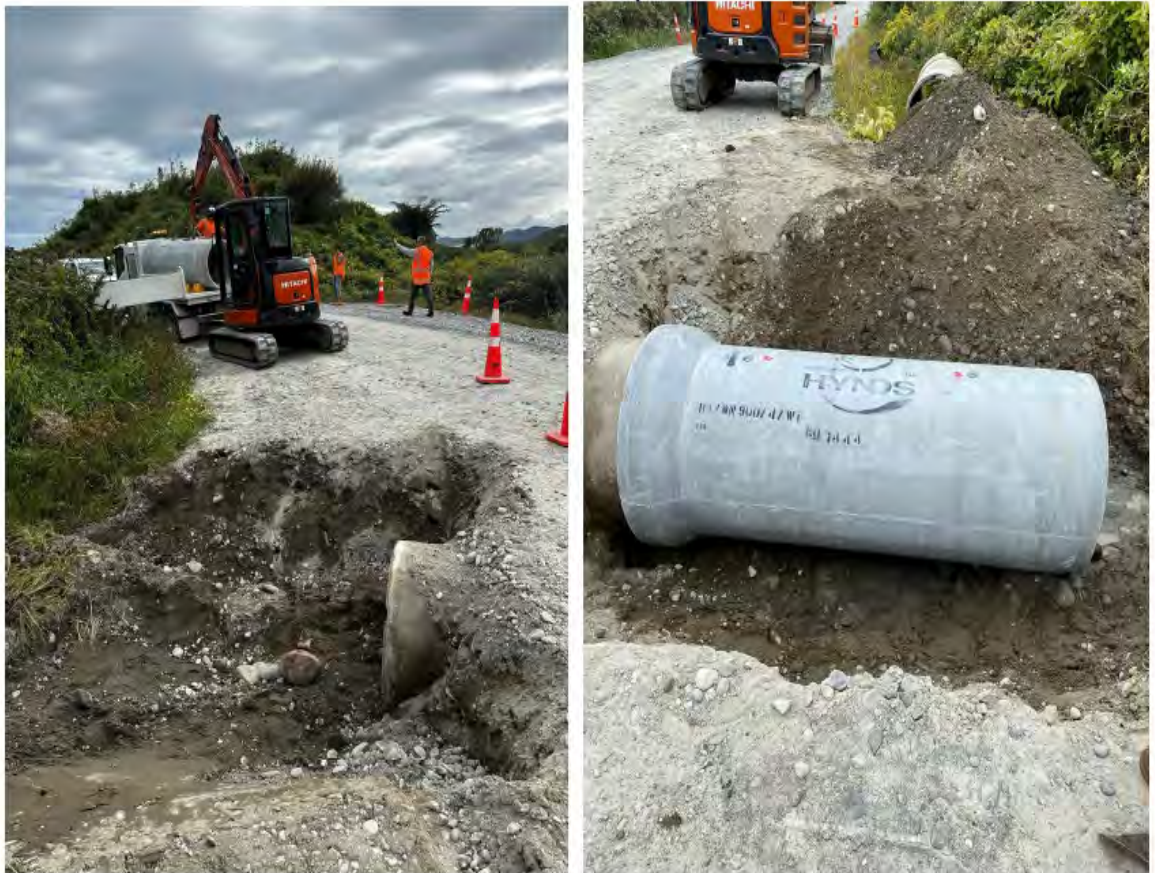
Figure 3: Culver Replacement on Domain Terrace Extension
