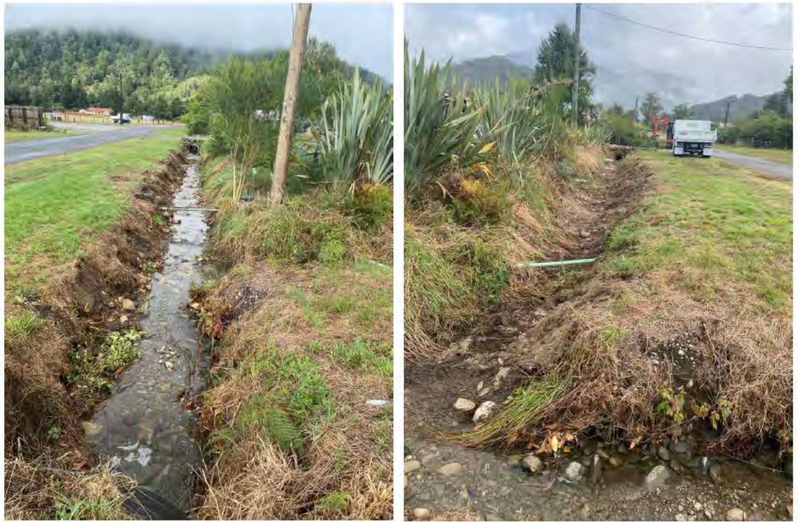
Figure 2: Blackball water table cleaning works
