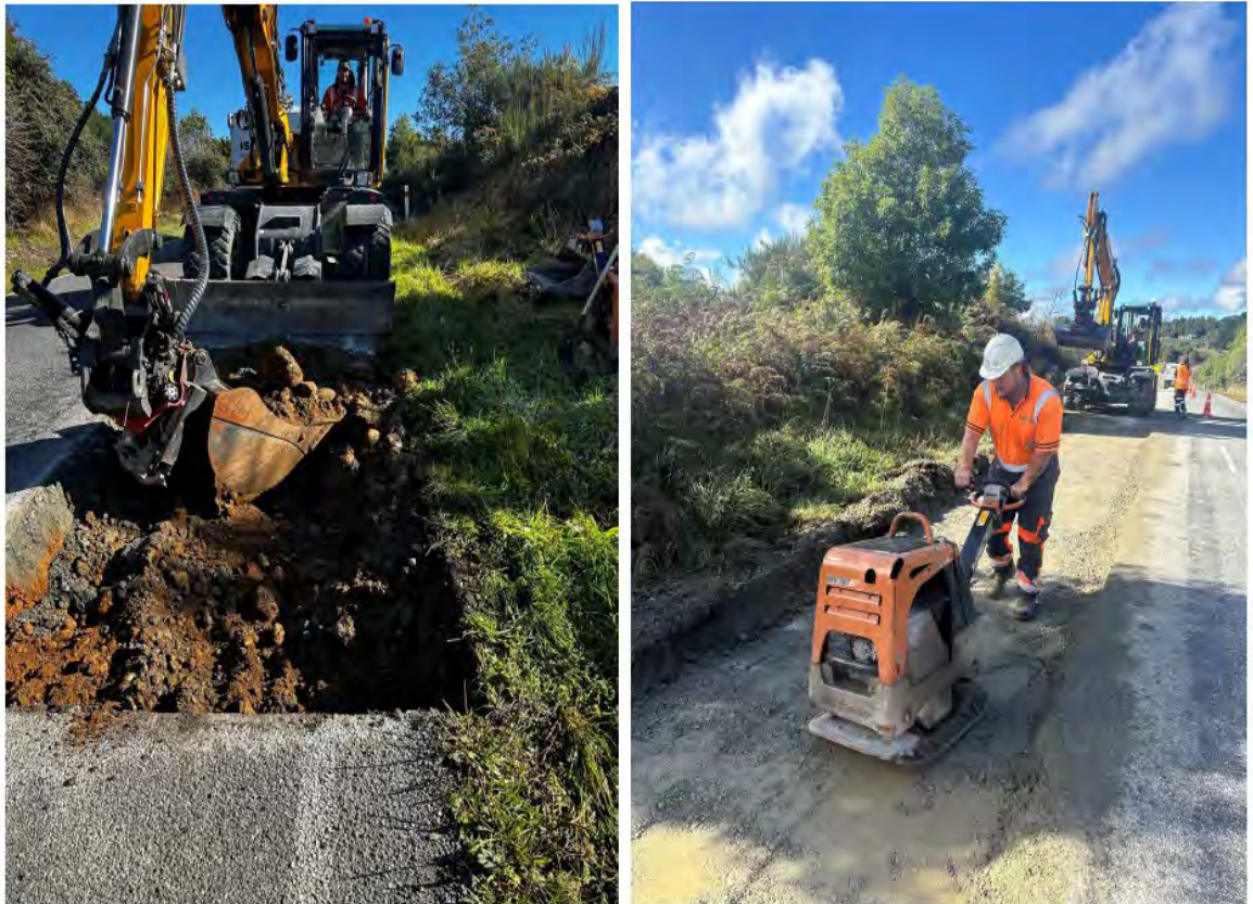
Fig 7: Pavement repair works on Arnold Valley Road
