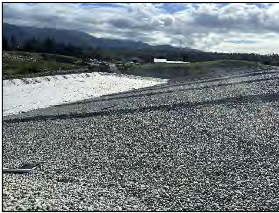
Fig 10 & 11: Photos showing the progression of liner layers being installed
