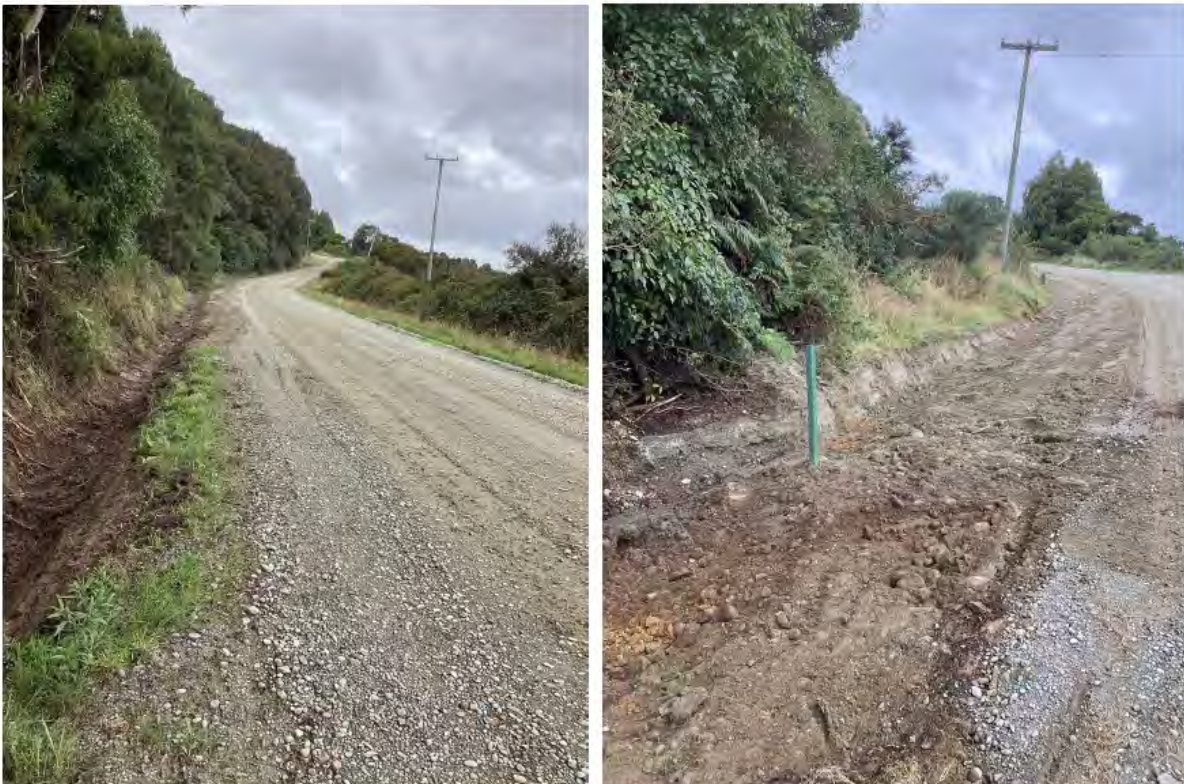
Fig 3: Drainage Maintenance works in Kotuku- Bell Hill Road
