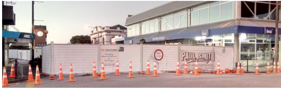
Construction site, Tainui Shared Street - April 2017
