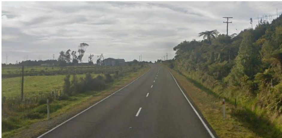
Figure 3: Existing Drainage Channel on SH6 Image Source: Google Streetview
