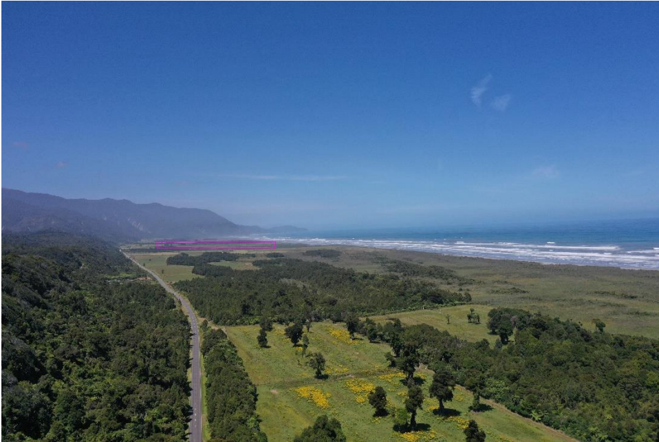
View from southern colony flightpath looking south at 100m elevation. The mining area is indicated in pink.
