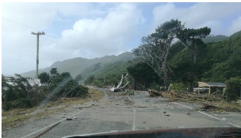
Photo 16. 01 Feb 2018 after ex-Cyclone Fehi, showing sea inundation just north of Fox River bridge
