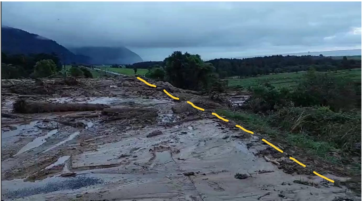
Photo 19. 09 May 2022 Landslide across road at Barrytown Flats, 3.3 kms south of proposed mine site. The yellow dotted line indicates the western road edge.
