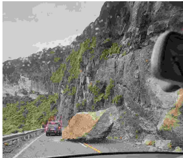
Photo 21. 30 July 2022 Rockfall above Waianiwaniwa / Ten Mile bridge
