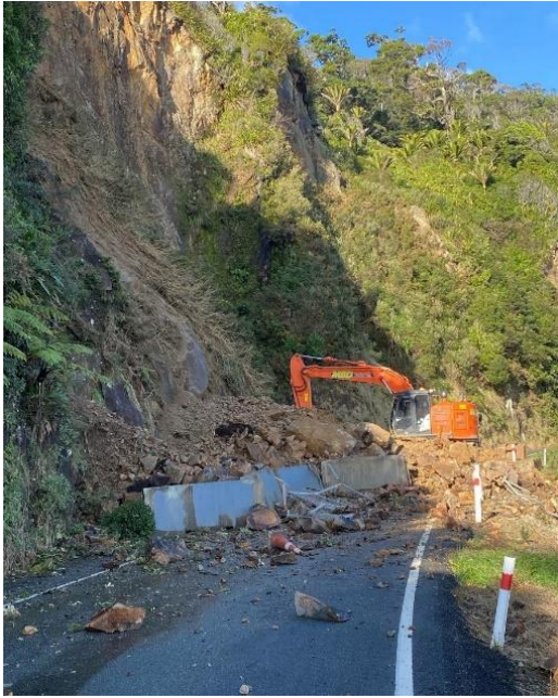
Photo 20. 17 June 2022 Meybille Bay, further slip closes road [following Sept 2016 slip which closed the road, then reduced it to one lane, as it remains today].
