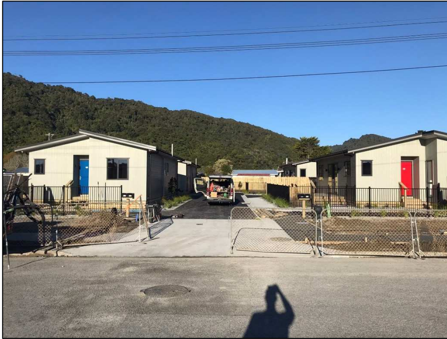
Photo of the new vehicle crossing and access
