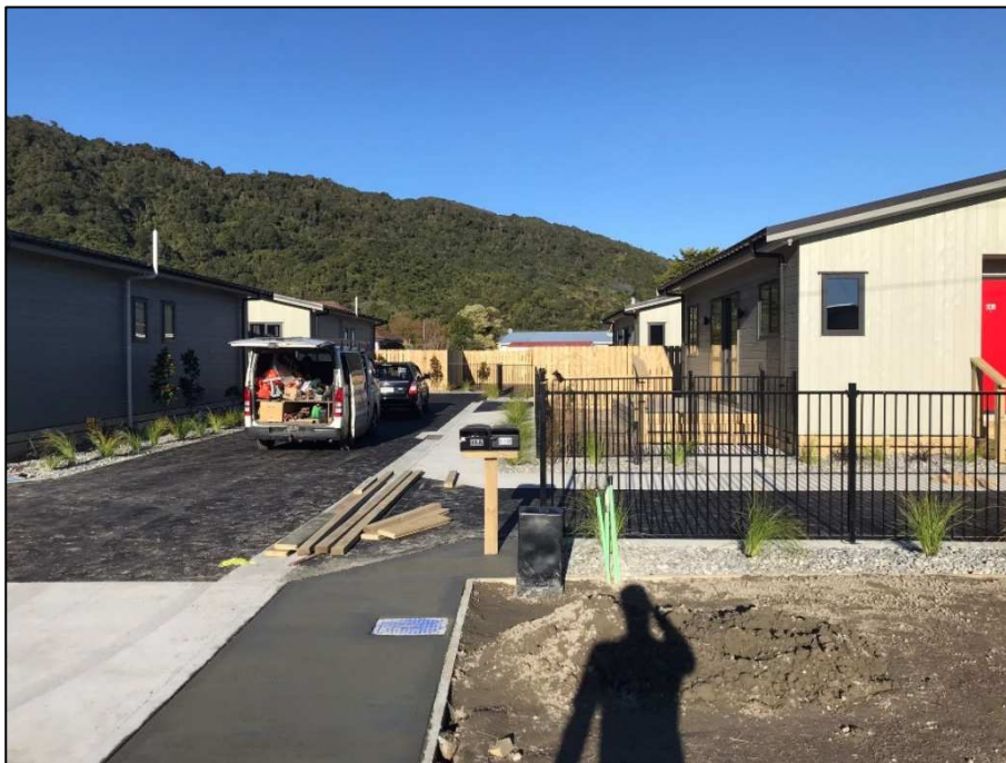
Photo of the new access
